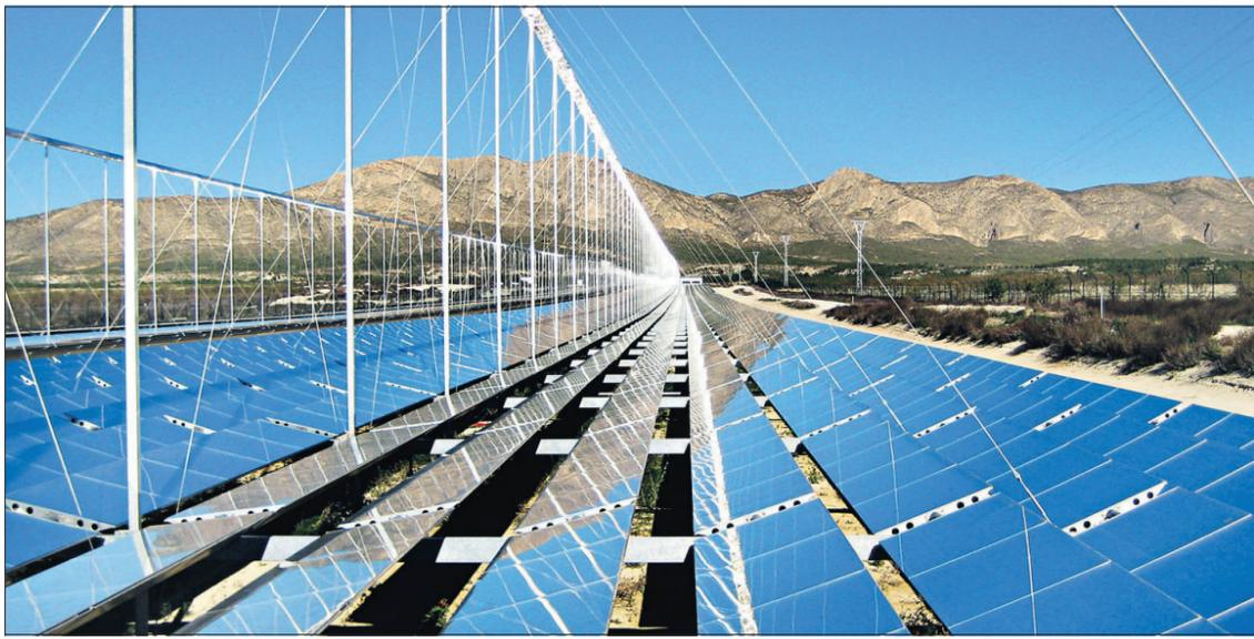
German company Novatec Biosol has developed a solar field using flat rather than curved mirrors, seen at its plant in Spain.
